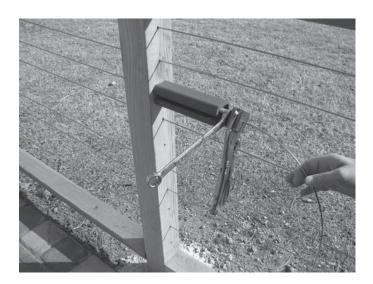
**4.** Using a ¾" wrench on the wrench flat of the all-thread, rotate the all-thread counter-clockwise, tightening the cable to the desired level of tension.
