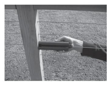
1. Place the pre-tensioner under the cable on which you plan to use it. Lift it up to the cable so the cable slips into the channel. The all-thread that extends beyond the housing should be facing the end post, with the back side of the pre-tensioner butted up to the next-to-last post/last intermediate post in the rail (not the end post itself).
