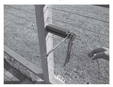
**4.** Using a ¾" wrench on the wrench flat of the all-thread, rotate the all-thread counter-clockwise, tightening the cable to the desired level of tension. Without having to pull tension through the entire cable, just from the pretensioner to the end post. When you have finished installing the cable at the end post, release the locking pliers, remove the pre-tensioner, and move on to your next cable, repeating the process.
