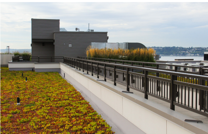
Alexan 100, modern architectural apartments, installed low maintenance aluminium Flat Top TR200 railing on common outdoor spaces.
