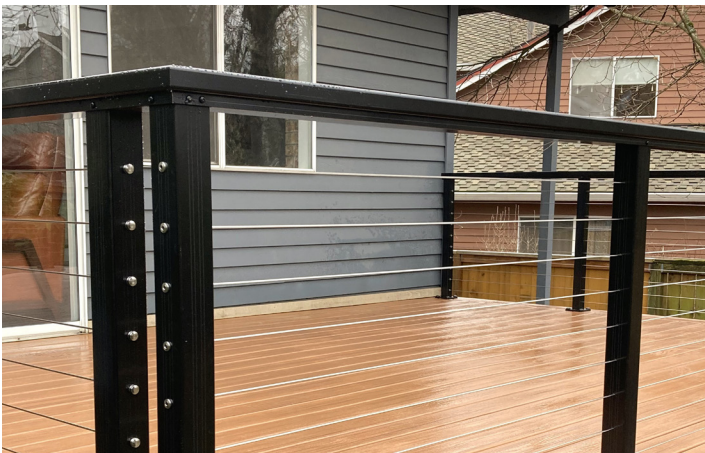
Stainless steel cable infill ensures safety and provides a seamless, unobstructed view, complementing the Flat Top TR200 railing on this backyard deck.
